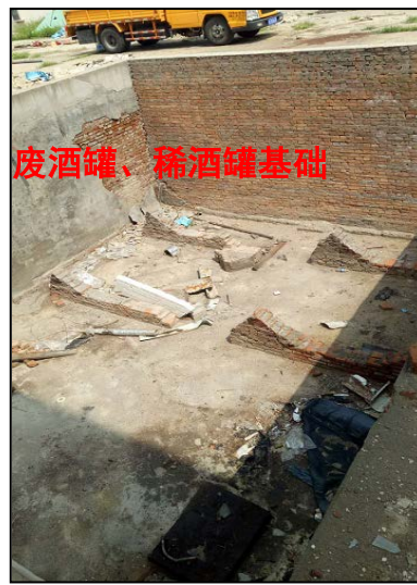
“浓酒罐”基础和“废酒罐、稀酒罐”围槽内有少量油污遗撒
